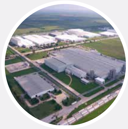
Manufacturing Plant, Lolita TX
